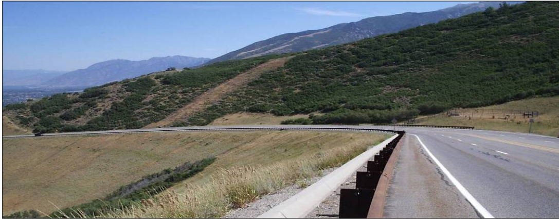
A portion of Traverse Ridge Road
